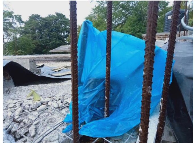
Fig -2: Place where the router place to have signal Source: Field data,2021
